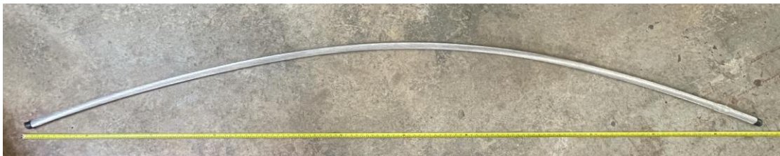
Figure 3-1: Image showing the approximately 13 foot length of the service exposed (used) conductor provided by NL Hydro as received for analysis.
